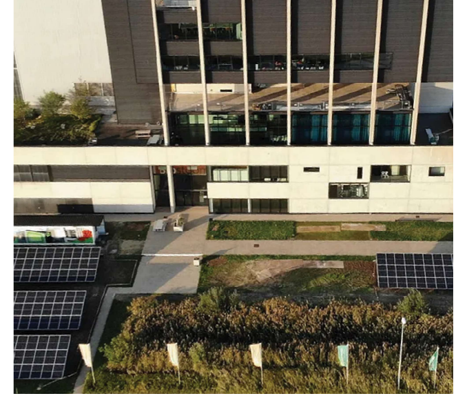
Circular Hub Bionerga Oostende
