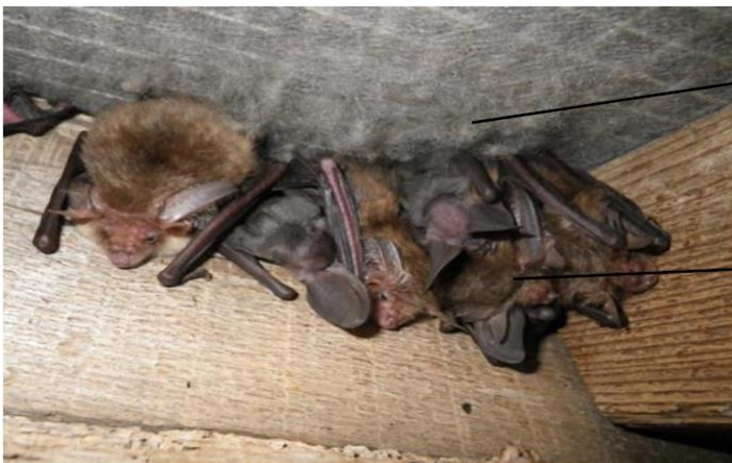
Figure 4. Example of fuzzing on a nonwoven membrane within a bat colony (Martin, Cumbria, UK)
