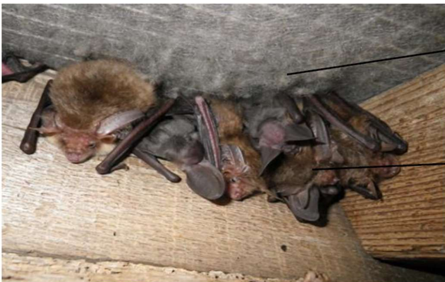
Figure 4. Example of furring on a nonwoven membrane within a bat colony Martin, Cumbria, UK)
