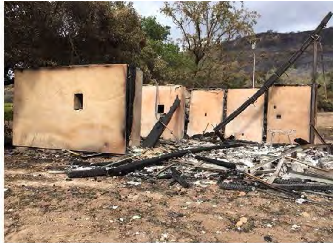
fig. 6. Napa Studio burned in the Atlas Fire; strawbale walls burned after the roof above was breached.
